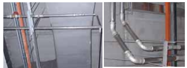
Internal Plumbing (Pipes install at ceiling)
